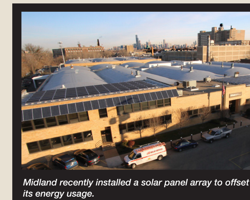
Midland recently installed a solar panel array to offset its energy usage.
